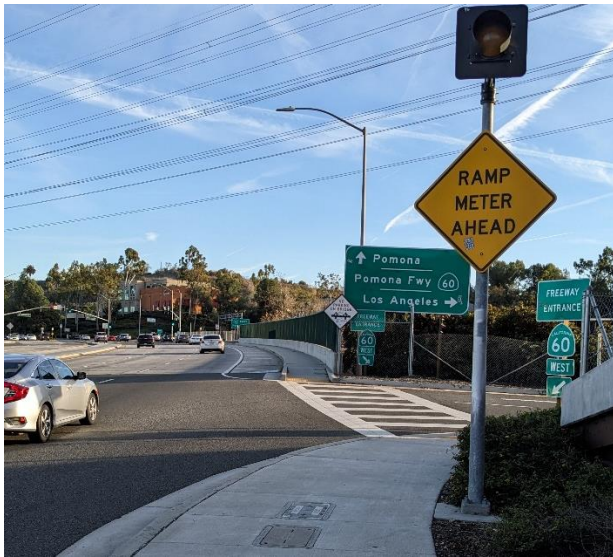
SR-60 RAMP AT PARAMOUNT BOULEVARD
