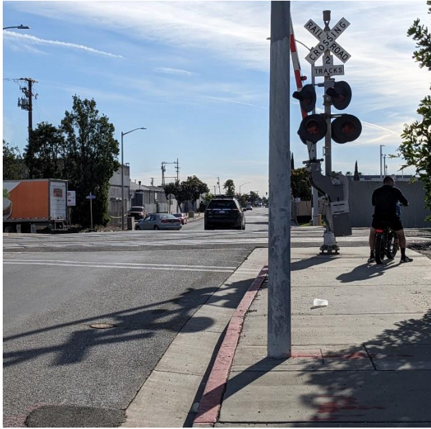
VAIL AVENUE RAIL CROSSING
